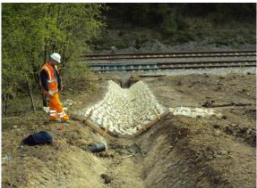
meant that the use of on-track plant to undertake the work wasn't feasible as the nearest RAP was a mile away from the worksite, therefore temporary access routes from the crest to cess level were formed to enable work to be undertaken using dumpers and midi-excavators in the cess. This method allowed us to utilise T2H possessions as an alternative to the lengthier process of booking T3 possessions.
