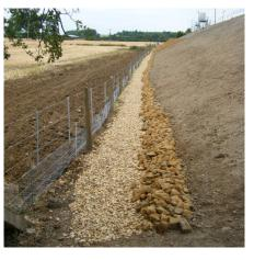
We were able to re-design the embankment crest works so that all work was carried out in fenced green zone working facilitated by installation of 500m of Vortok fencing and the use of small plant.
